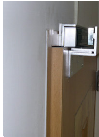
Installation of the Armature for Electromagnetic Lock
