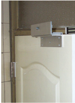
Installation of the Armature for Electromagnetic Lock
