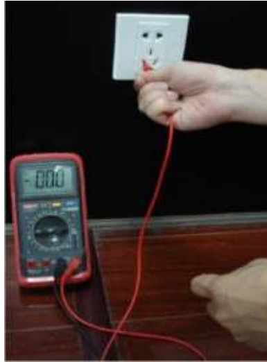
Appendix Figure 7-7 Check neutral cable connection
