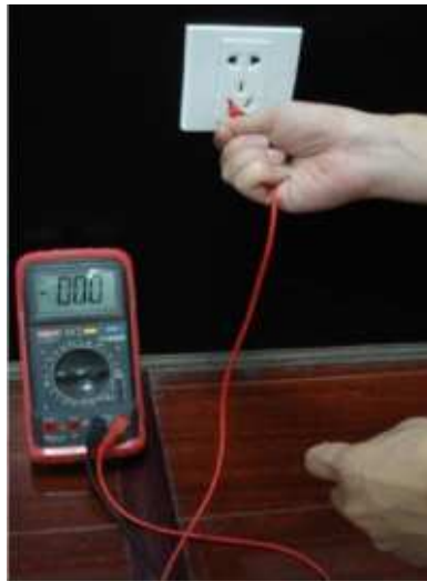
Appendix Figure 7-7 Check neutral cable connection
