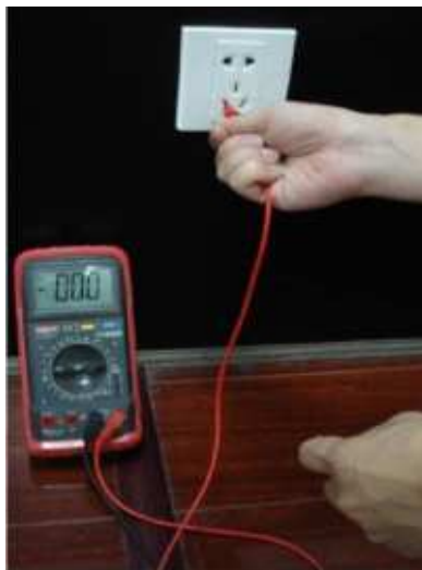
Appendix Figure 7-7 Check neutral cable connection
