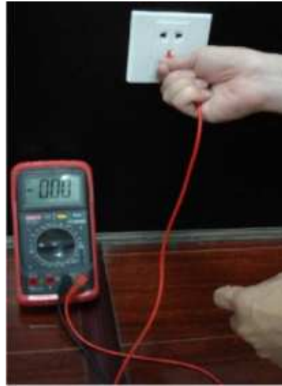
Appendix Figure 7-5 Check earth cable connection
