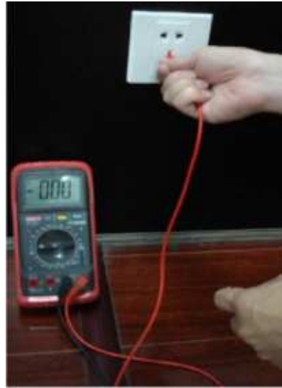
Appendix Figure 7-5 Check earth cable connection
